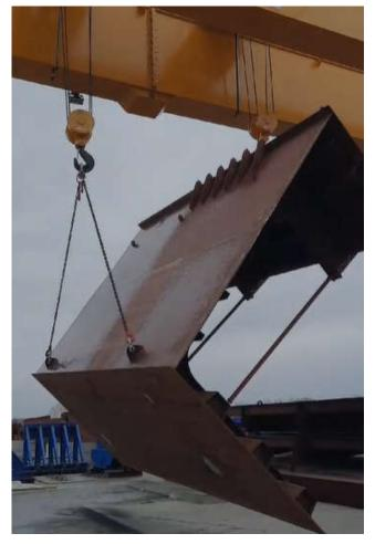
The block modules arriving at the project site were combined into blocks in the gas submerged arc welding building temporarily established on the site, and placed on the platform for block assembly before incremental launching process.
