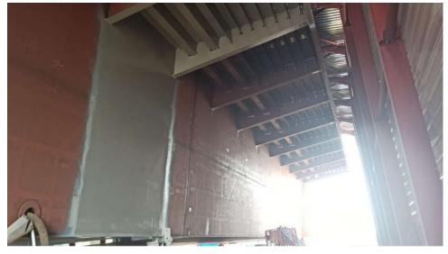
Sandblasting and anti-corrosion protection coating were performed for the assembled block in the paint building temporarily established on the site.
