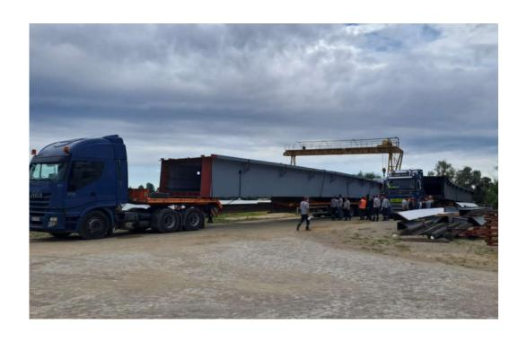
Due to the carrying capacity of the bridge transportation block dimensions, the modules and consoles were transported separately and the assembly works were carried out at the preassembly site in Belgrade. 7 blocks, whose preassembly and touch painting works were completed and ready for final assembly, were transported to the project site by barge over the Sava River and assembled on temporary piers by lifting of floating crane.
